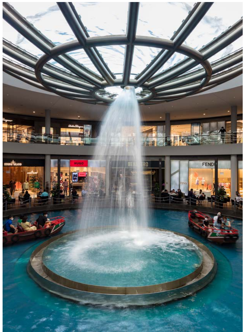
The Rain Oculus functions as both a skylight and a rain collector, where up to 22,000 litres of water flow through every minute.
